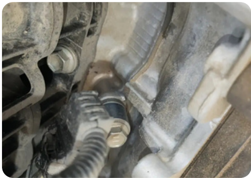
Engine Exterior: Signs of leakage present
